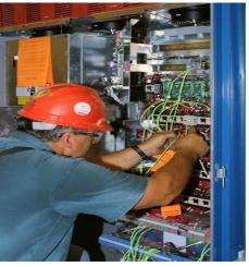
Relay logic or PLC control wiring and panels must be restored including partially rewiring, replacement of microcircuitry and sensitive relays, contacts and din rails prior to being tested and put back into service. It is important that professionals work on these technical aspects of the claim from beginning to end to ensure that the systems are inventoried, restored, tested and put back into service with track ability.
