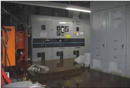
***Flooded main gear and power distribution system in high rise building***
